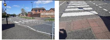
A barrier fence runs along the zig-zag markings on both sides of the school front gate to add additional safety.
